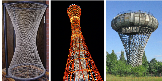
FIGURE 3. Hyperboloids “in the wild.” From left to right: A hyperboloid model, a hyperboloid at Kobe Port Tower, Kobe, Japan, and cooling hyperbolic towers at Didcot Power Station, UK. These are all examples of quadric surface scrolls with a double ruling.
